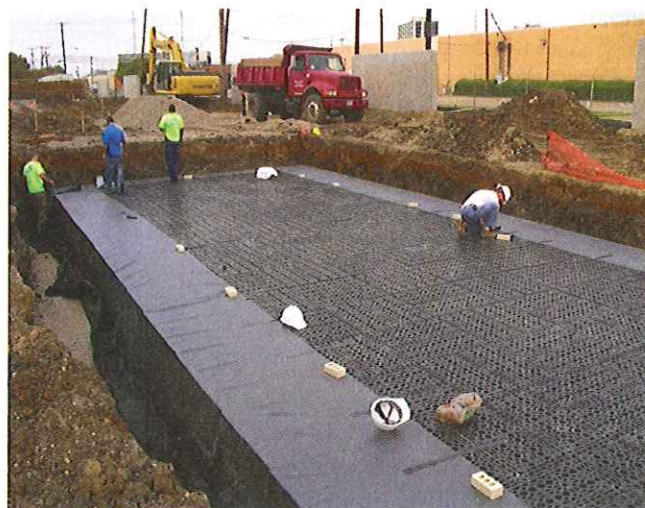
Left: Workers place the tanks in the excavated area. Right: The liner and fabric was pulled up and over the tanks while another sheet of liner was placed on top of the system and glued in place.
