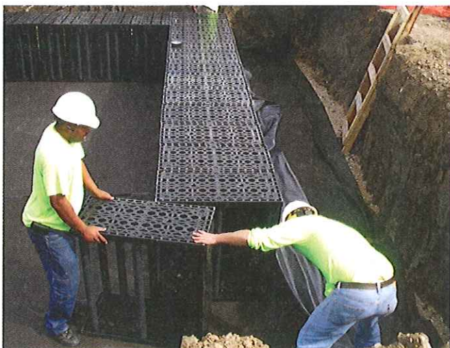
Left: Workers place the tanks in the excavated area. Right: The liner and fabric was pulled up and over the tanks while another sheet of liner was placed on top of the system and glued in place.
